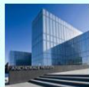
Anchorage Museum Anchorage, Alaska
