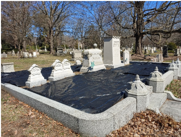
Figure 3 – Fortunately, the use of black plastic for covering smaller defined areas within curb and fence lots for several months to kill weeds and weed seeds has proven to be successful.
