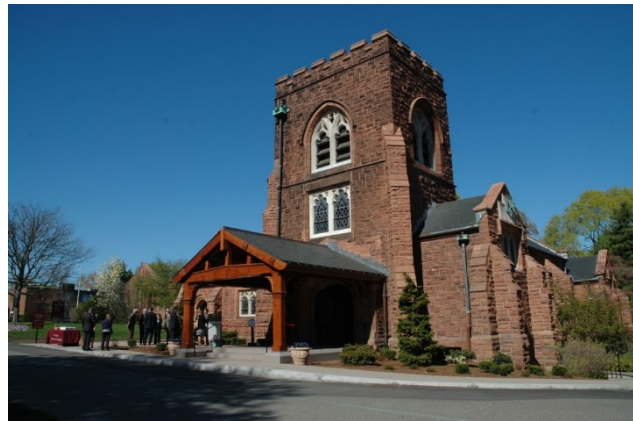
Figure 1 - Story Chapel's new front entrance is now more welcoming and accessible. The new entryway was rebuilt with beams purchased from a salvage lumber yard in Connecticut.
